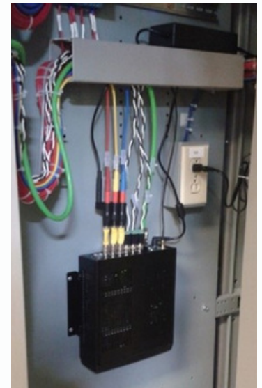
The I3CM 5G FL can be fixed with the provided fixation brackets. Illustration of this type of fixation.
